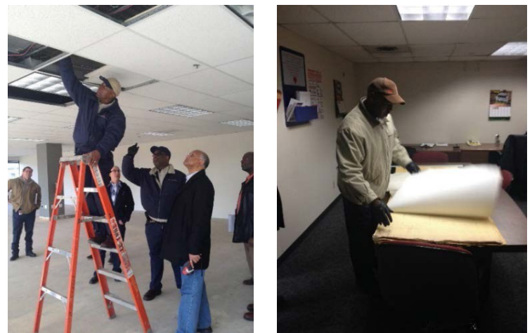
Figure 4. Building walk-down included checking above the ceiling for duct condition, etc. (left) and reviewing electrical and mechanical prints (right)
