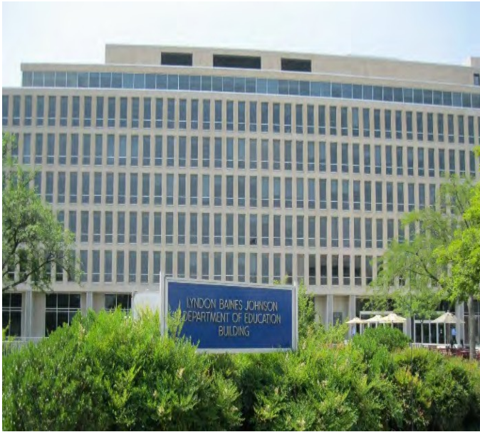
LBJ Department of Education Building Address: 400 Maryland SW, Washington, DC 20202 Owner: U.S. General Services Administration Size: 550,800 Rentable Square Feet
