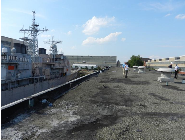
Figure 28 Roof of Building 669
