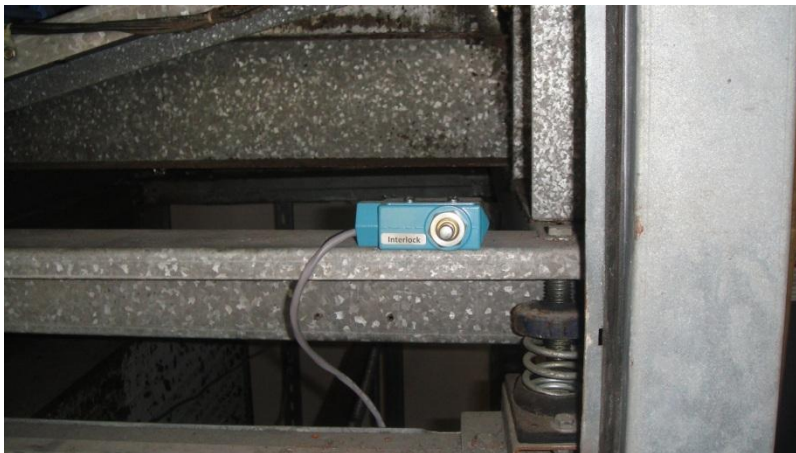
Figure 4 – UV lamp interlock with door
