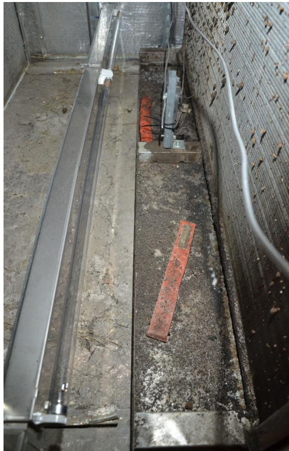
Figure 6 – UV lamps and downstream side of coil
