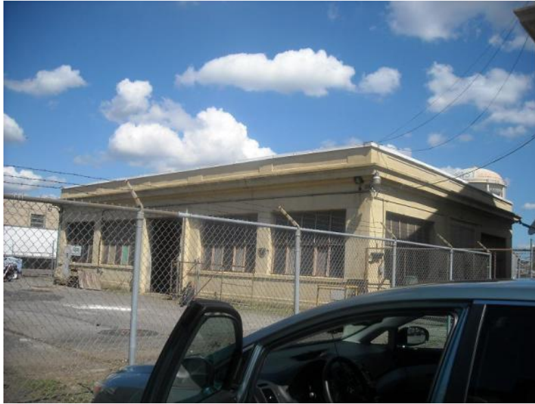
Figure A.69.1: Front entrance of building 69
