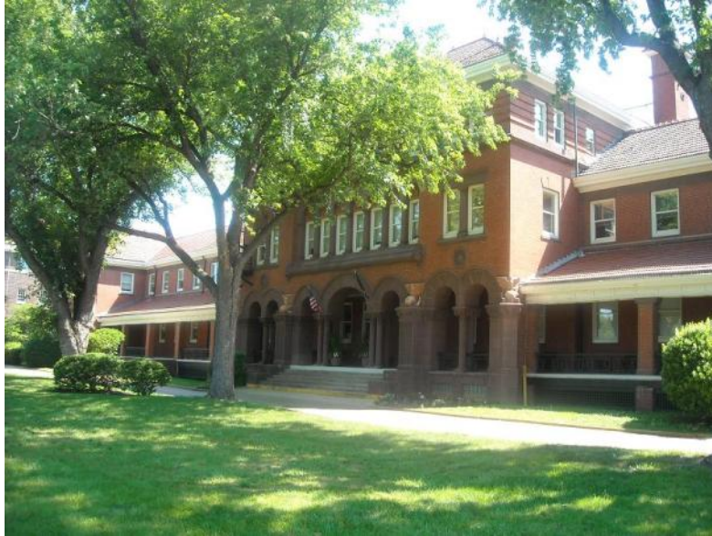
Figure A.100.1: Front entrance of building 100
