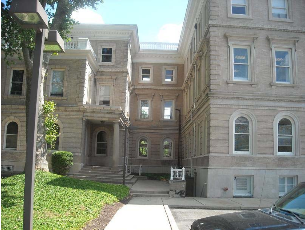
Figure A.6.1: Rear of building 6 showing complex planform shape
