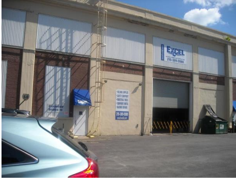
Figure A.68.1: Front entrance of building 68
