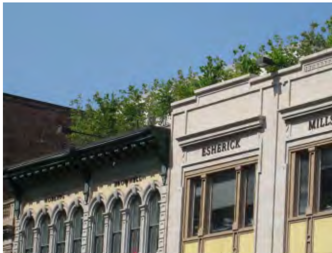
Figure 6 | Example of incompatible green roof treatment from the National Park Service 32
