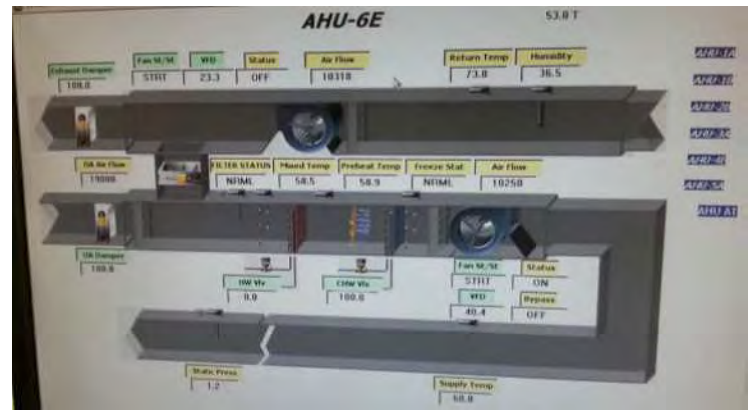
Figure 7. AHU economizer damper commands and temperature sensor data
