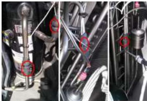
c) Thermistors along Refrigerant Loop      d) Air Temp Probes & RH sensors
