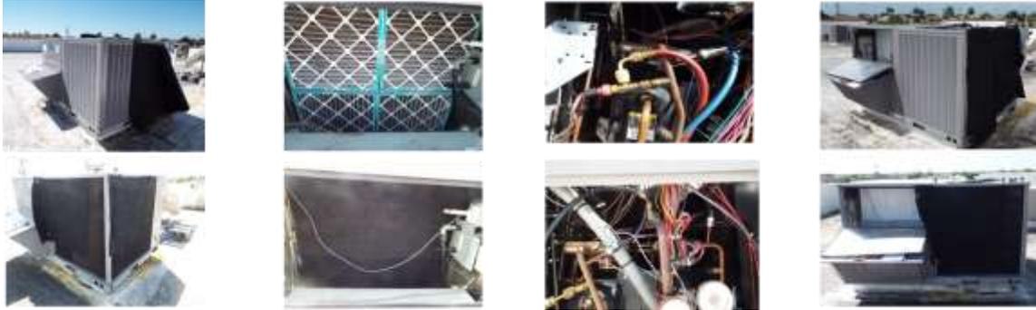
a) Condenser Blockage      b) Evaporator Blockage      c) Compressor Bypass      d) Cond. & Evap. Blockage
