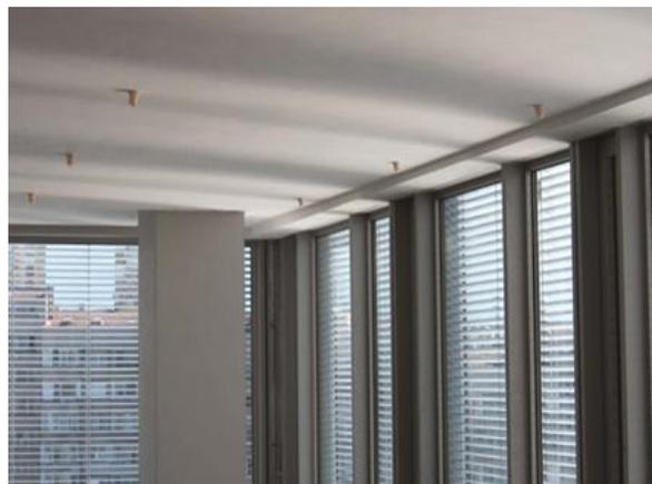
Figure 24 Light redirecting blinds maximize daylight contribution (Koester, 2012)
